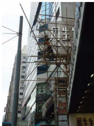
Worker erecting bamboo scaffolding in Hong Kong
